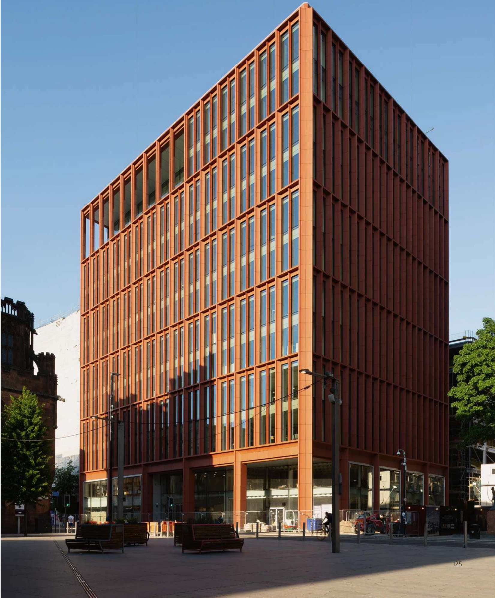
LINCOLN HOUSE, 125 DEANS GATE, MANCHESTER, UK. ARCHITECT: GLENN HOWELLS, LONDON
